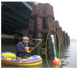
Fig. 05. A 6" PVC pipe is embedded 20 feet deep and attached to the side of this piling containing a YSI 6000 series DO sensor.
